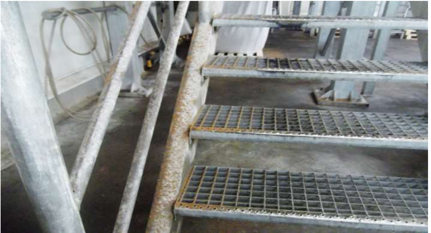
Fig. 2. Poultry meal deposited on the galvanized steel constructions can not be easily differentiate from iron rust.
