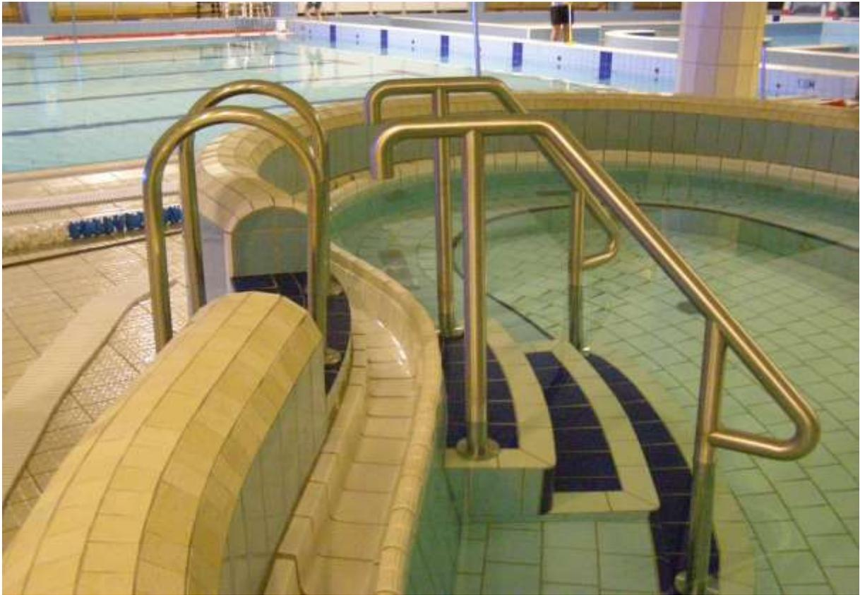
Fig.3. 316L stainless steel railings situated out of the air streams washed every day did not show any corrosion signs
