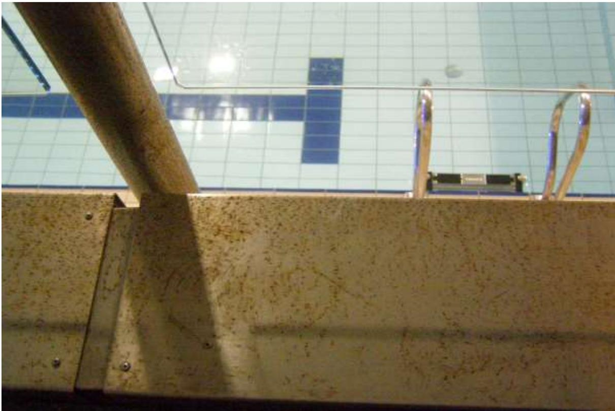
Fig.2. Aerosol of chlorine compounds carried by air stream to the ventilation air exits effected corrosion of stainless steel plates and railings at the terrace
